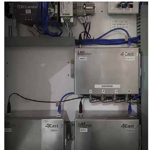
—The sensors are connected to the 4Cast, a central processing unit with internet connection.
